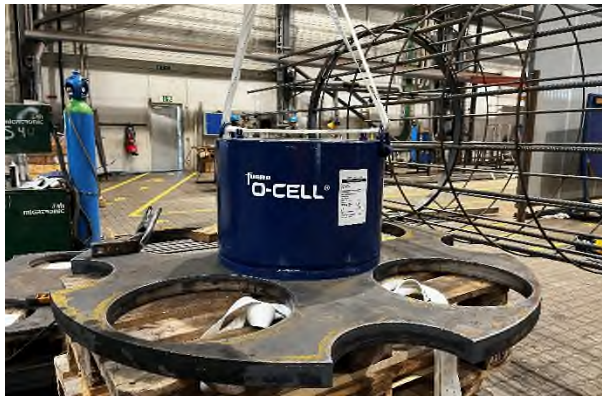
O-Cell assembly preparation and installation
