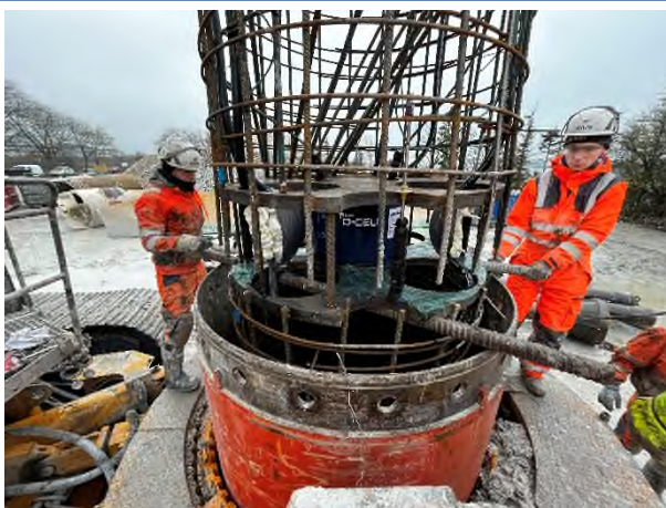
O-Cell assembly final preparation
