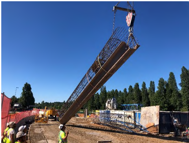
Reinforcing cage lifting
